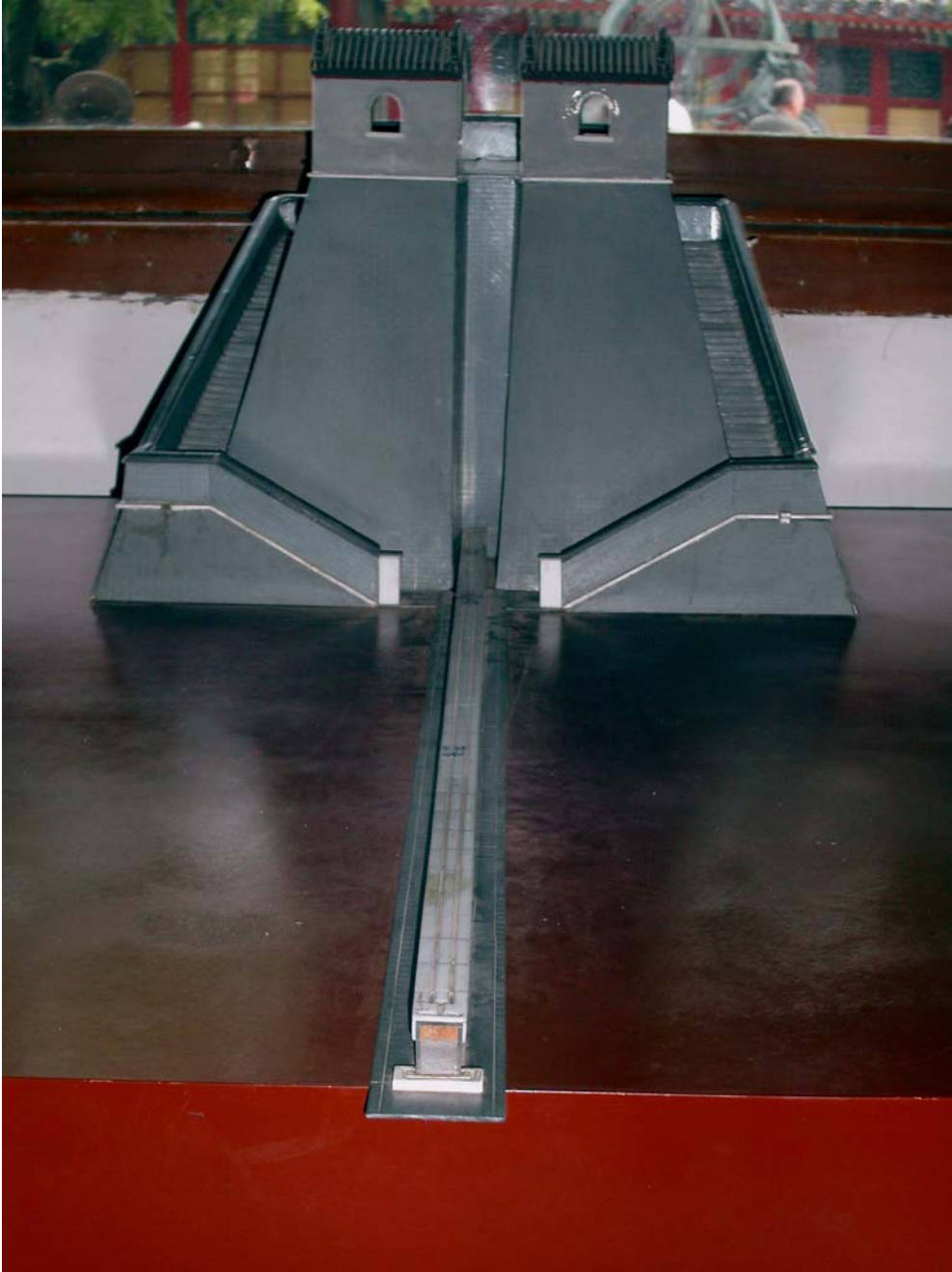
Figure 1. Model of Dengfeng Star Observation Platform designed by Guo. The actual platform is 31 feet tall with a path for measurements extending 105 feet in front. This monumental instrument with Guo's innovative shadow aligner allowed more precise measurements than were possible with the smaller gnomons.
